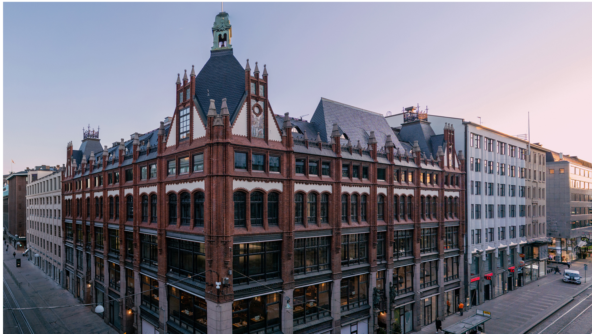
Aleksanterinkatu 13 renovation of office premises, Helsinki, Finland
