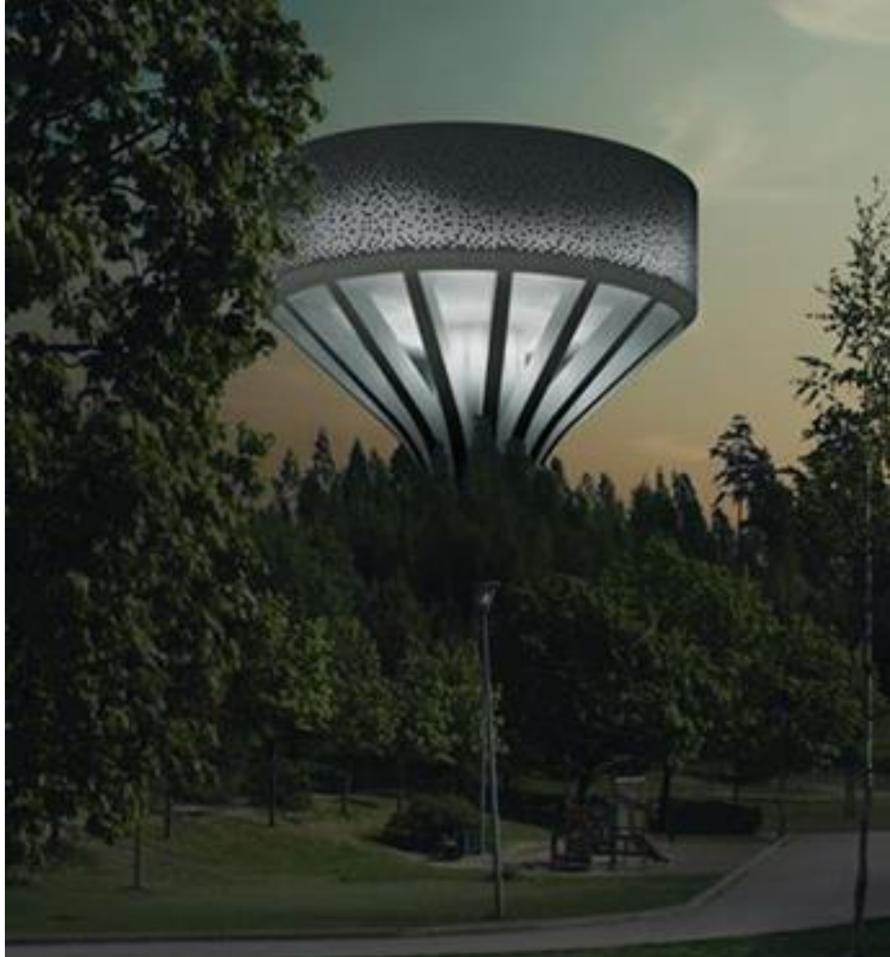
Hiekkaharju water tower Vantaa, Finland
